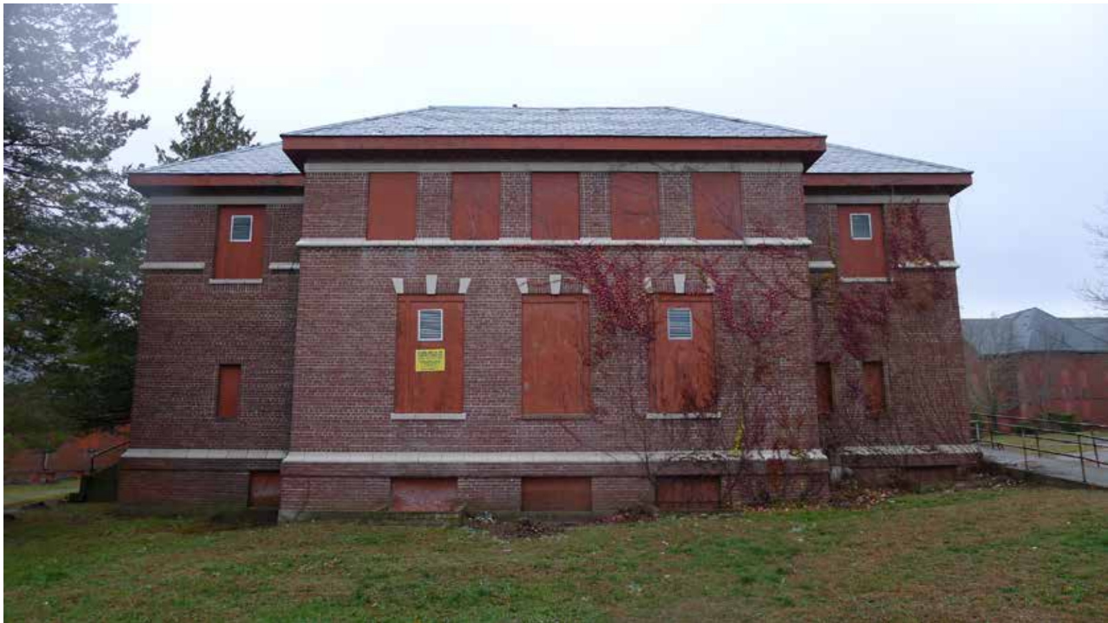
Figure 35. South elevation of Infirmary
