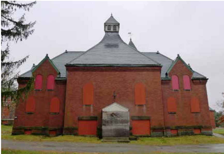
Figure 20. North elevation of Lee Hall
