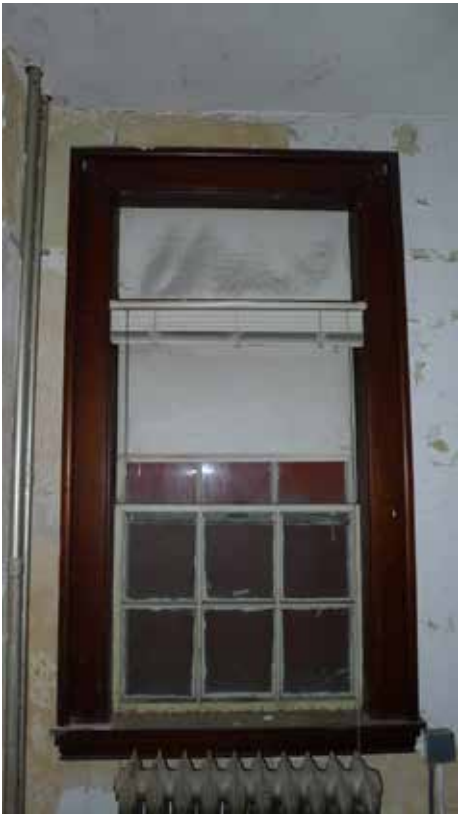
Figure 14. Typical double-hung window
