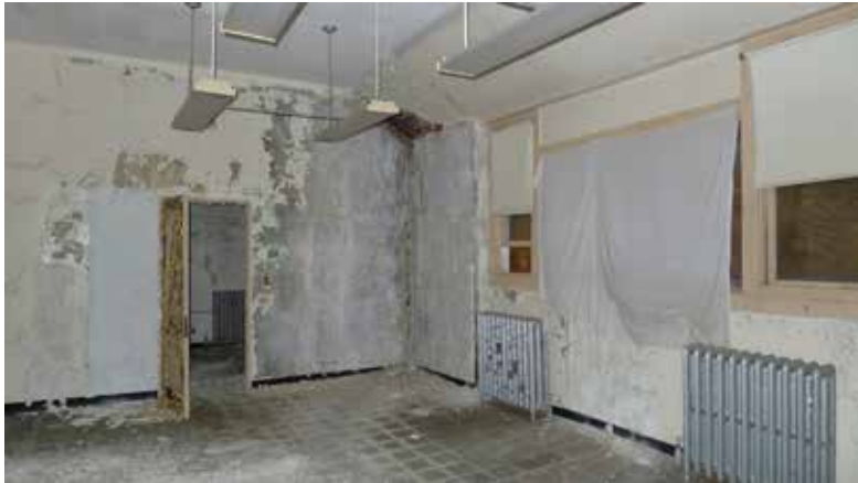
Figure 39. 3rd floor - south room
