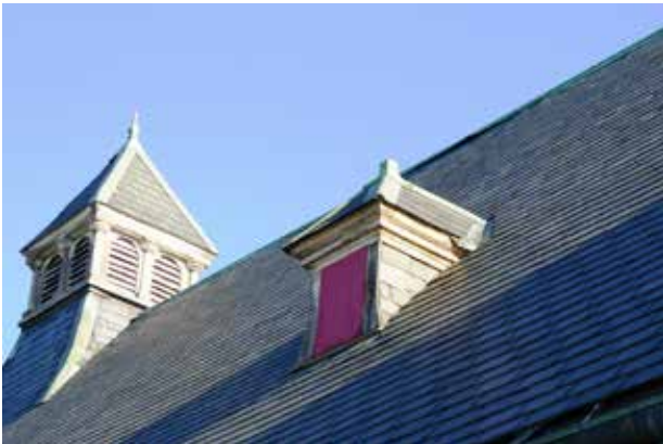
Figure 21. Slate roof, cupola and dormer
