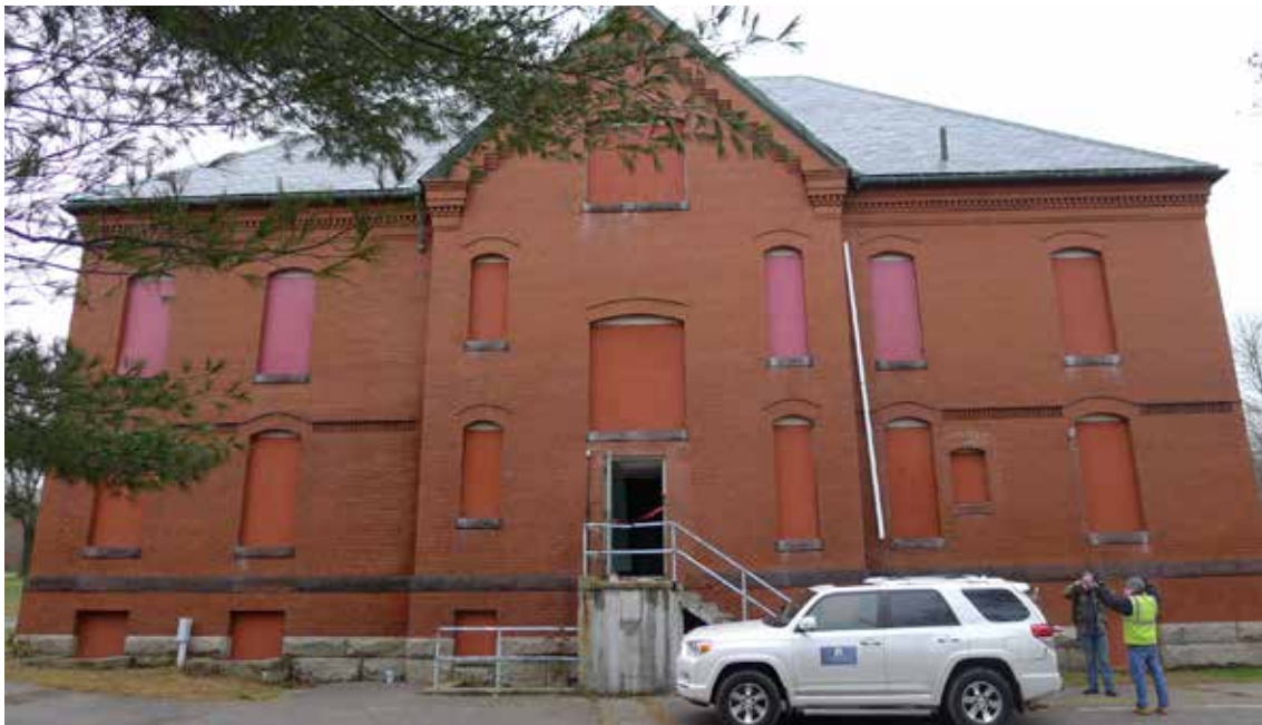
Figure 5. West elevation of building #22A Administration.
