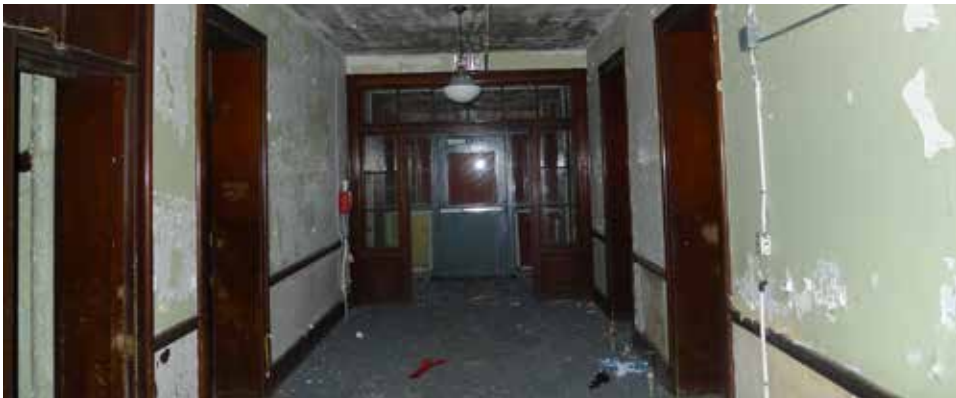
Figure 12. 1st floor hallway - looking north
