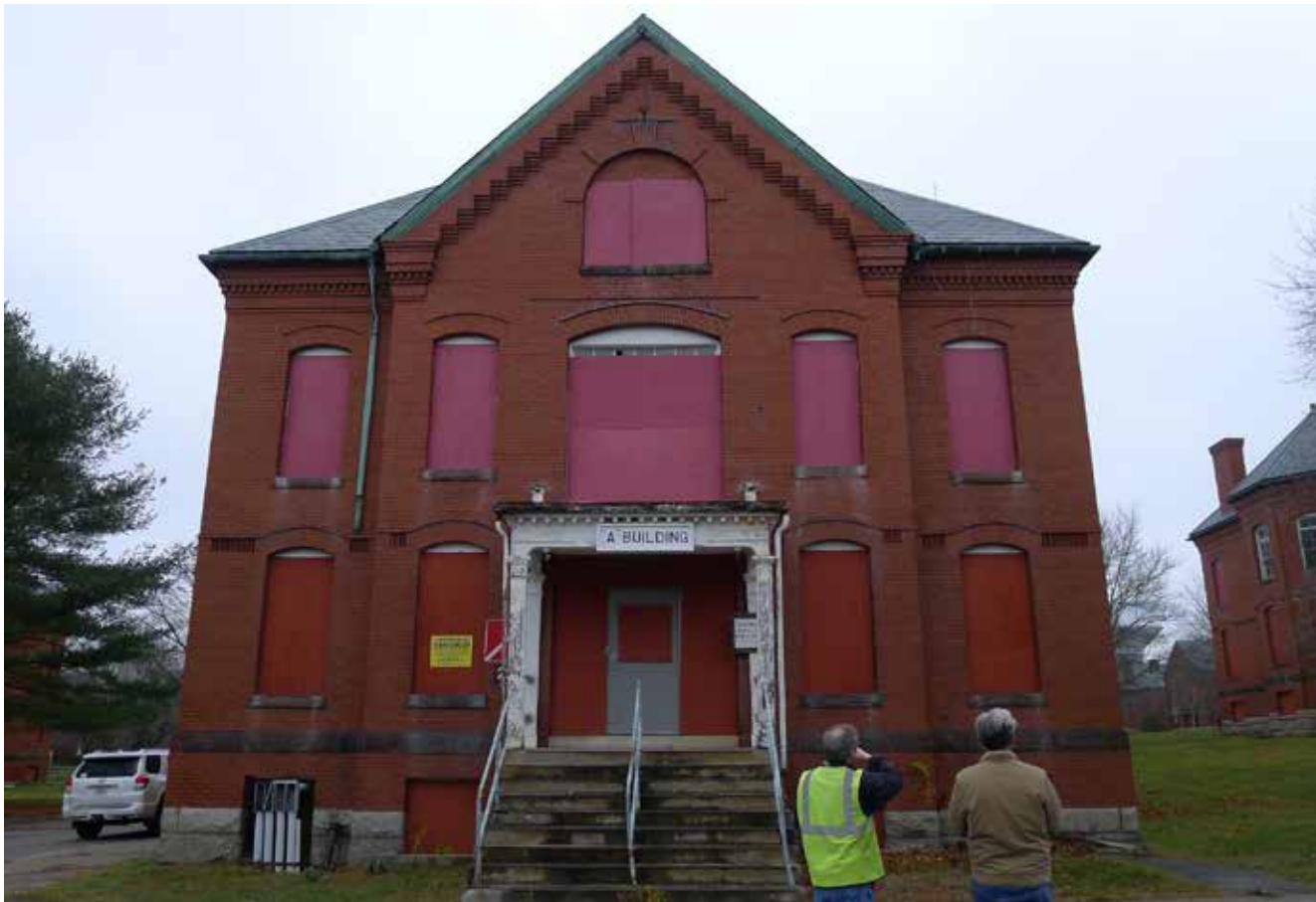
Figure 3. South elevation of building #22A Administration.
