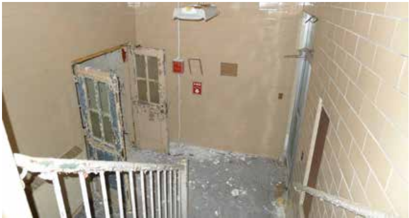
Figure 45. East stairway (non - original)
