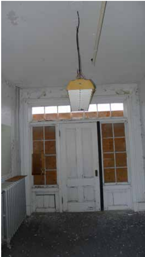
Figure 7. 1st floor entry door looking south
