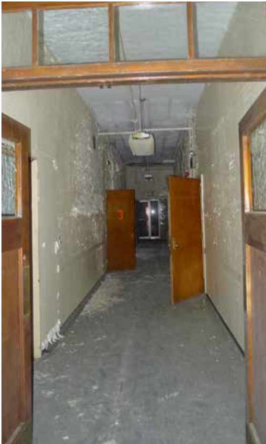
Figure 40. First floor corridor - looking west
