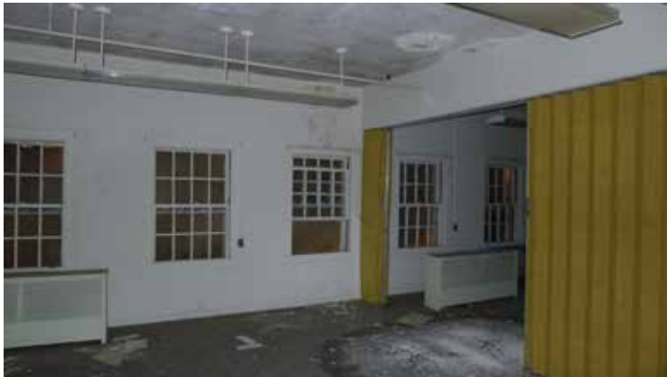
Figure 41. 3rd floor large room
