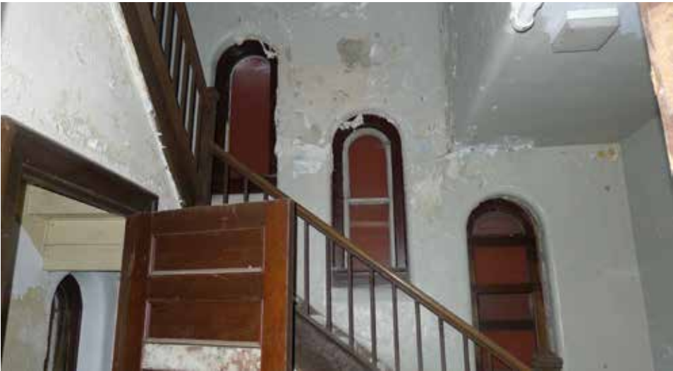
Figure 32. Replacement and original windows - southeast stair
