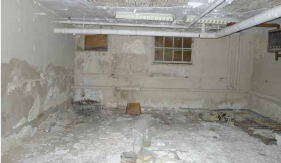
Figure 48. North room in basement
