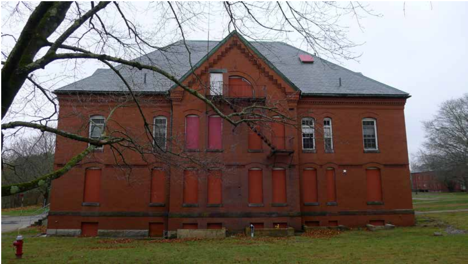
Figure 4. East elevation of building #22A Administration.
