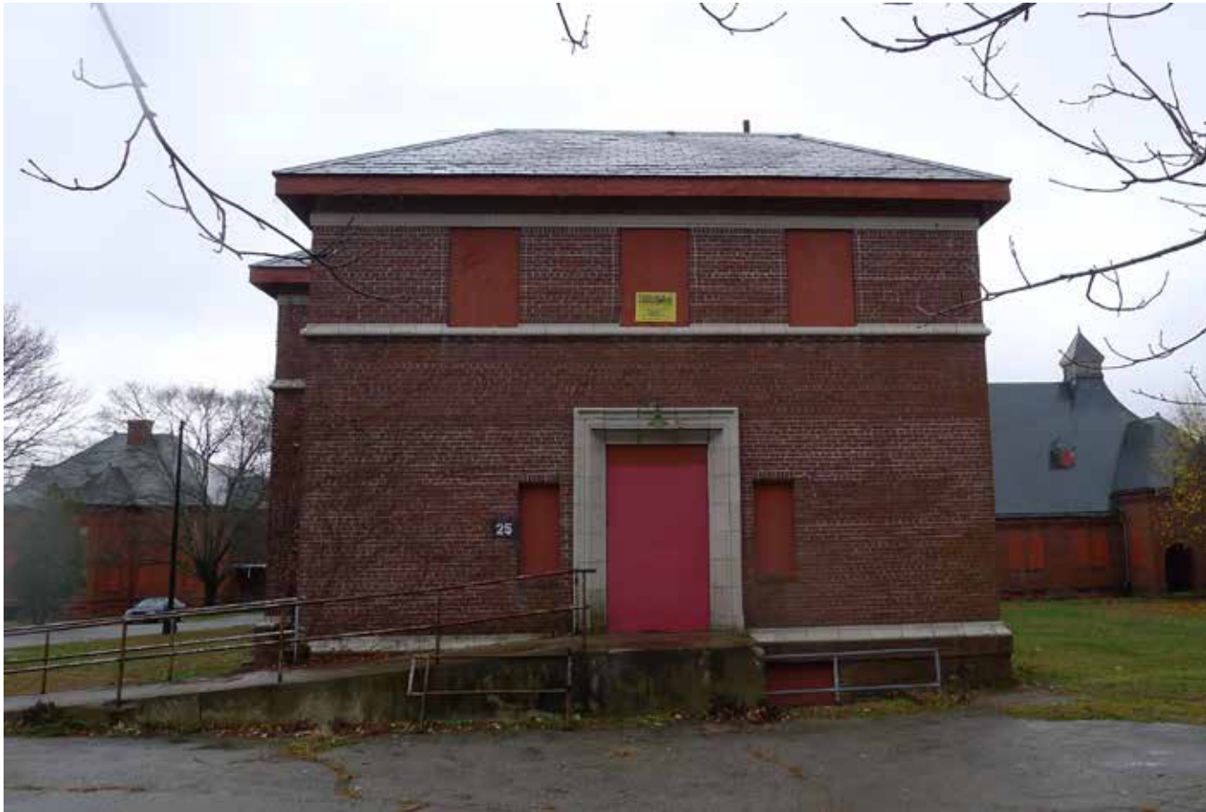
Figure 34. East elevation of Infirmary
