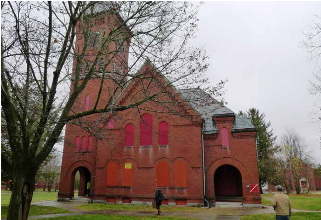
Figure 17. South elevation of Lee Hall
