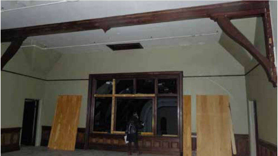
Figure 31. Formal balcony mezzanine - looking south
