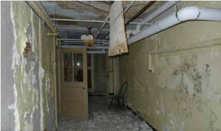
Figure 42. Basement - central hallway looking west
