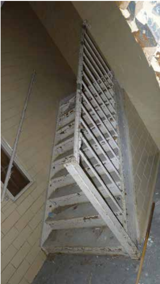
Figure 46. East stairway (non - original)
