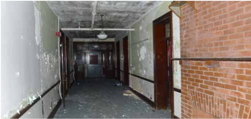
Figure 11. 1st floor hallway - looking north
