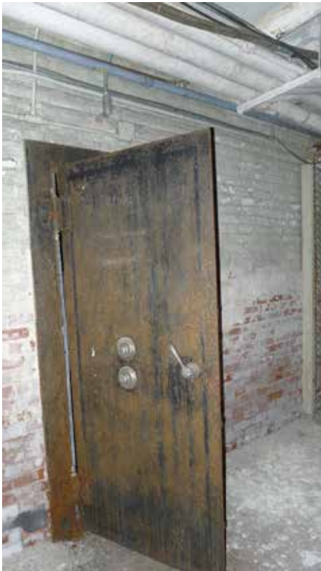
Figure 13. Vault door - basement
