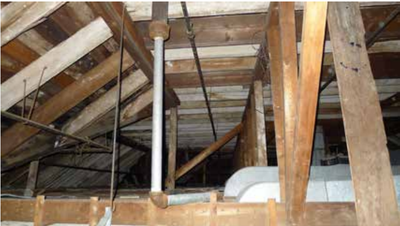
Figure 44. Wood roof framing - attic
