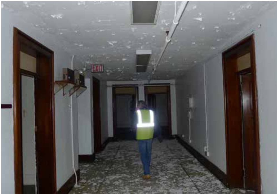
Figure 15. Third floor hallway - looking south
