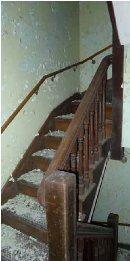
Figure 9. Secondary stair first floor landing
