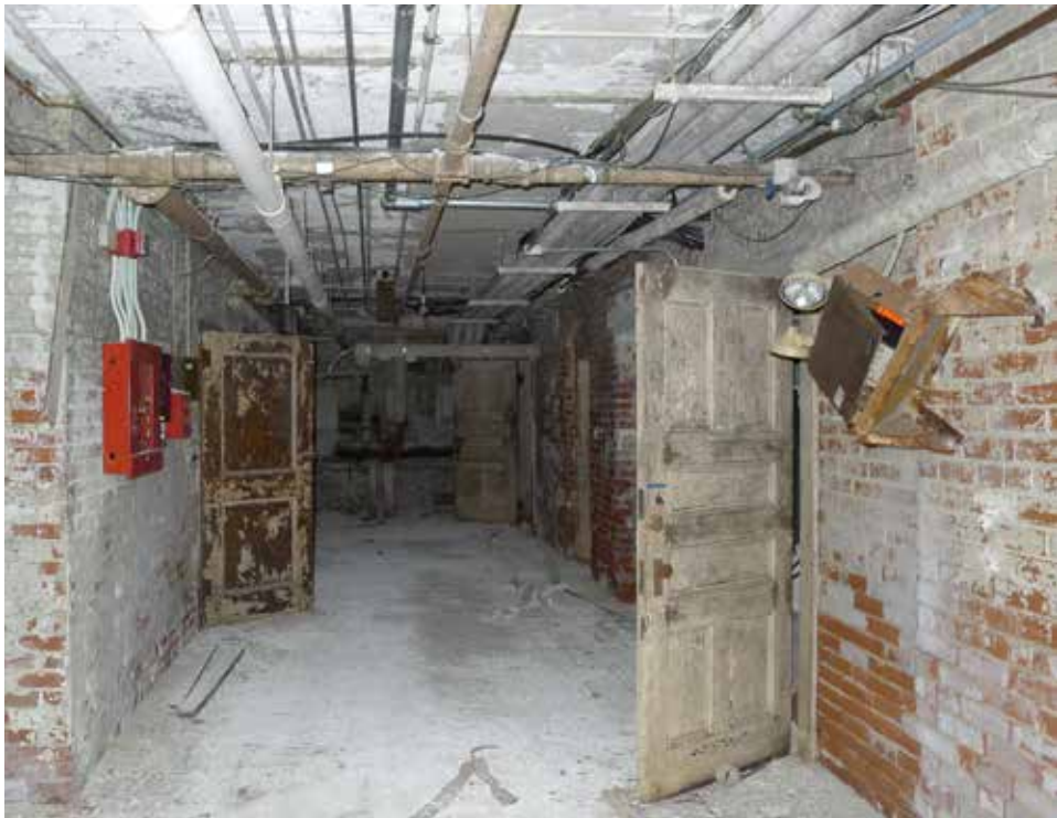
Figure 16. Basement hallway - looking south
