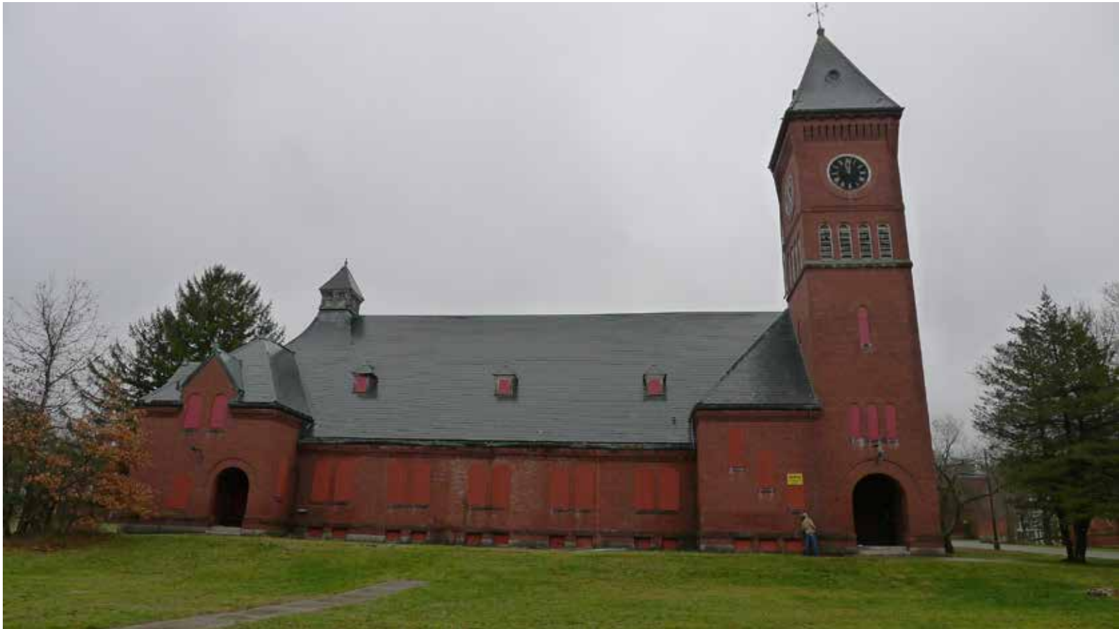
Figure 18. West elevation of Lee Hall
