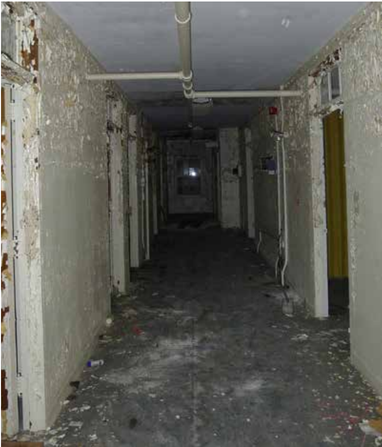
Figure 43. 2nd floor central hallway looking west
