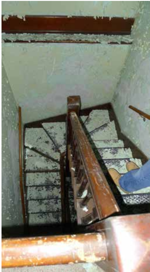
Figure 10. Secondary stair to basement
