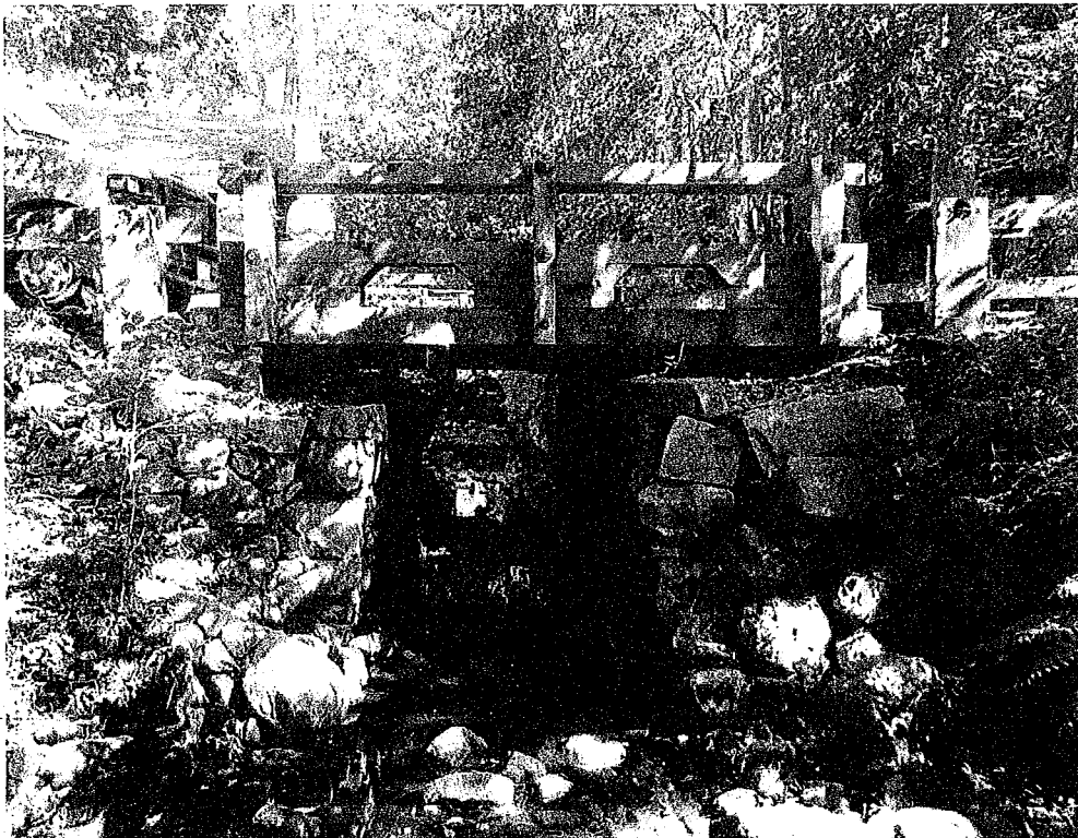
Photo 6: Proximity of the abutments to the channel walls.
