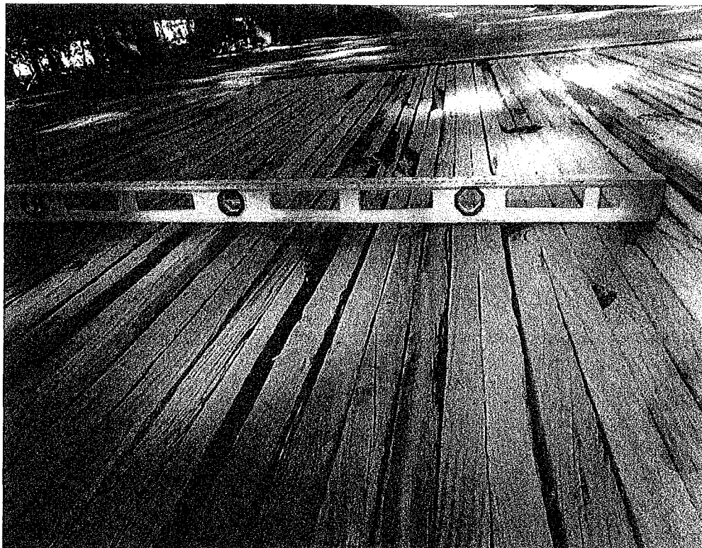
Photo 1: One inch of sag and crushing at joint of panels 2 & 3.
